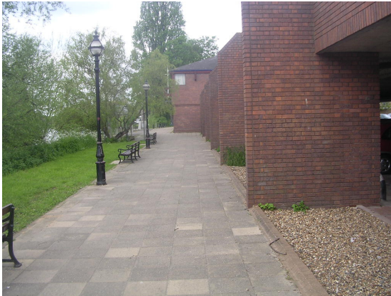
Plate 1: View along Thames side path, Car Park on right. The sea cadet building can be seen at the end of the path.
