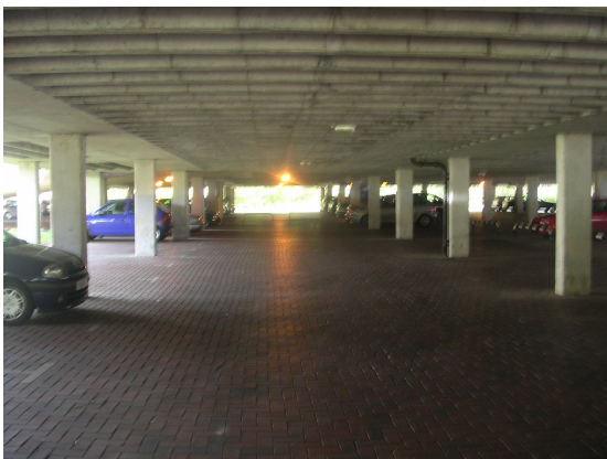
Plate 3: View through Car Park, ground floor
