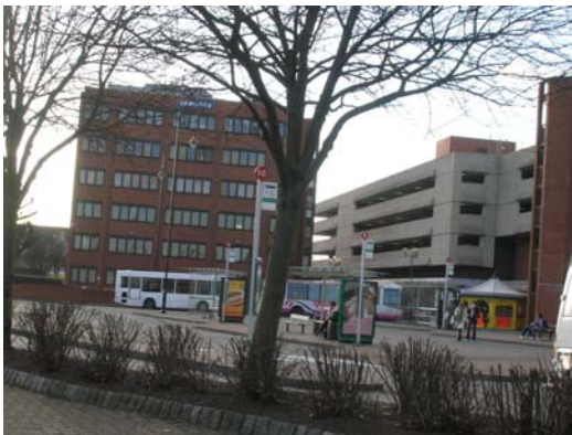
Plate 1: View towards bus station and Communication House
