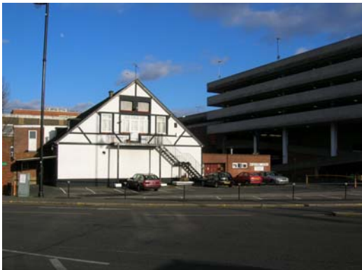
Plate 3: Hall in Western extension area
