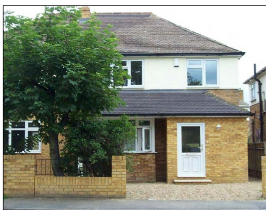
Front extension to semi-detached property with roof form to match main roof
