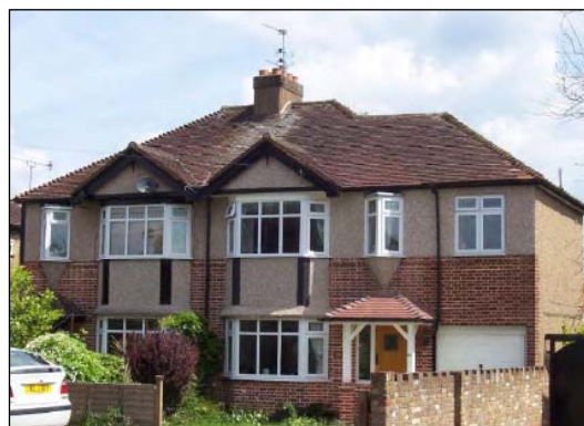
Example of a well designed side extension
