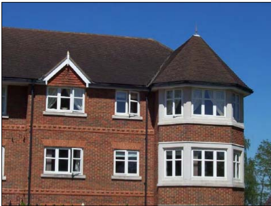
Roof, brick and stone detailing
