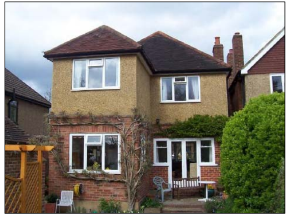
Subordinate two storey rear extension
