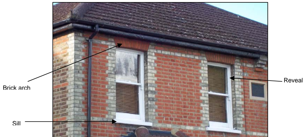
Diagram 9: Components of a window and opening
