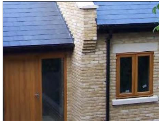
Brick, stone and lead detailing
