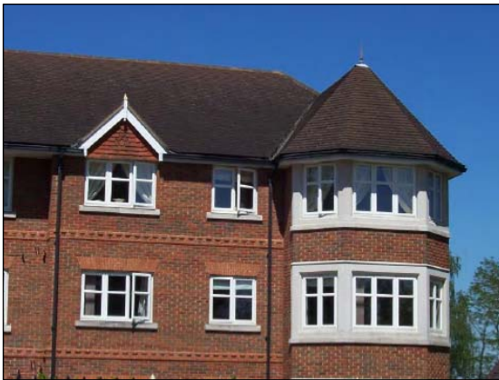
Roof, brick and stone detailing
