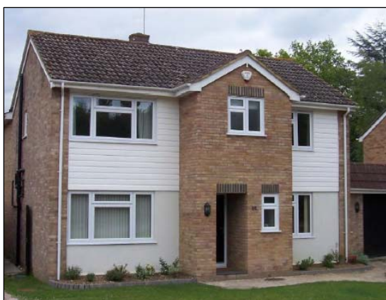
Balanced front extension to a detached property
