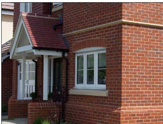
Brick and stone detailing
