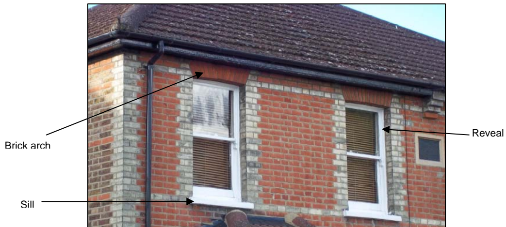
Diagram 9: Components of a window and opening
