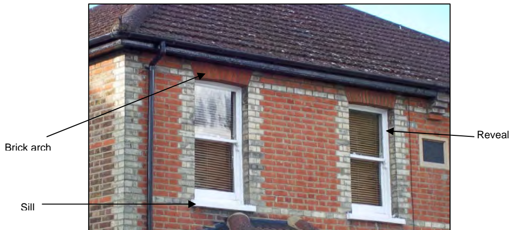
Diagram 9: Components of a window and opening
