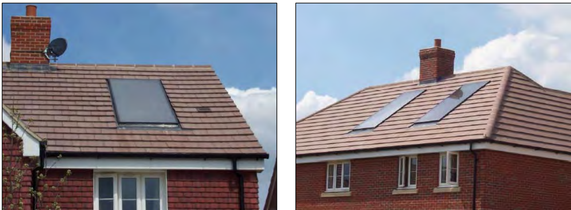
Flush mounted solar panels
