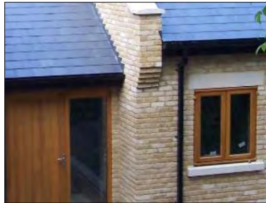
Brick, stone and lead detailing
