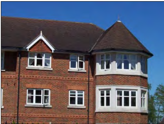
Roof, brick and stone detailing
