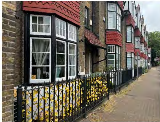
Sunbury-on-Thames - detailed facades
