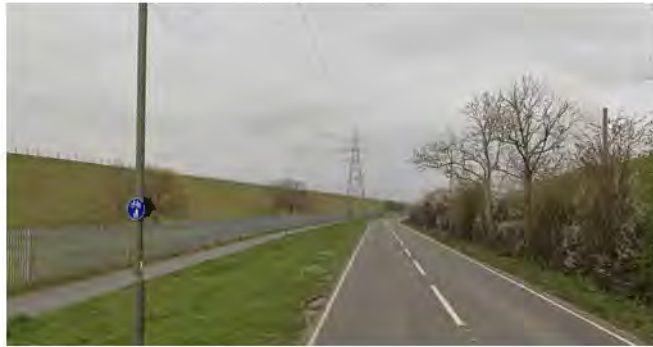
Embankments between Staines Reservoirs
