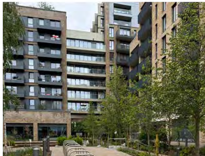
Development at approximately 350dph (Staines)
