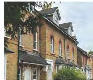
Dormer windows and brickwork detailing
