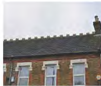
Roof decoration and prominent chimneys
