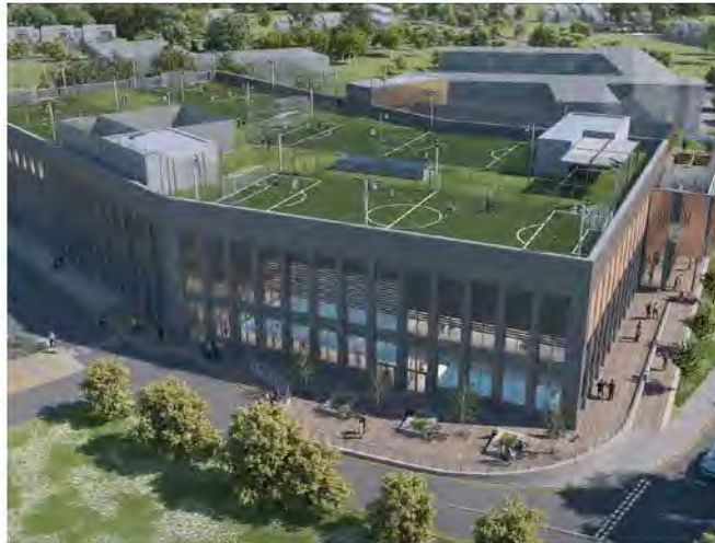
Spelthorne Leisure Centre (under construction)
