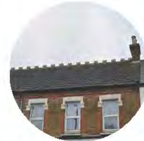
Victorian roof features
