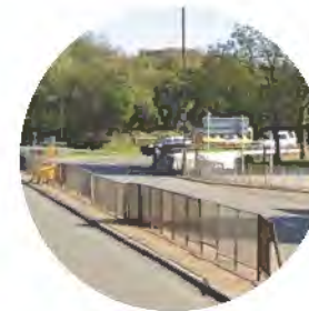
Railings causing severance
