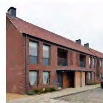
Inset balconies on maisonette upper floors
