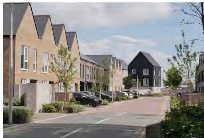
Marker building terminating view along street
