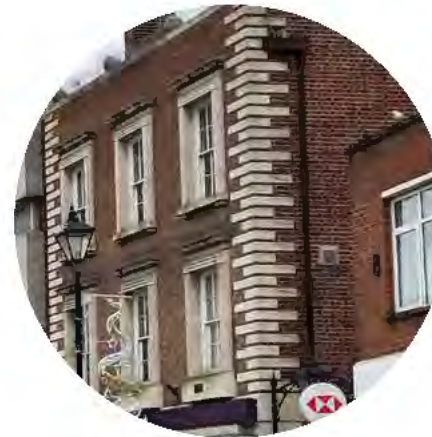
Corner brickwork detailing and brick variation
