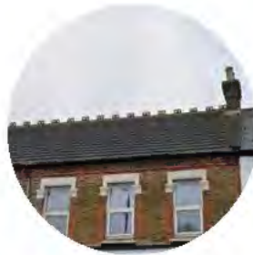
Roof line features
