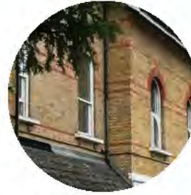
Changes in brickwork
