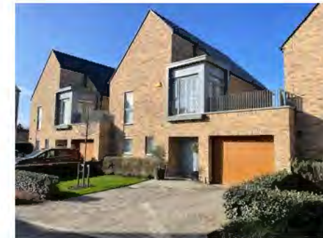
Integrated garages and roof terrace design
