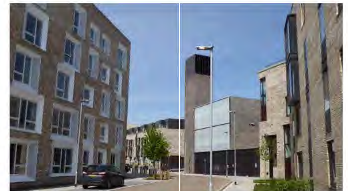
Energy Centre co-located with supermarket fridges and designed as marker building in street
