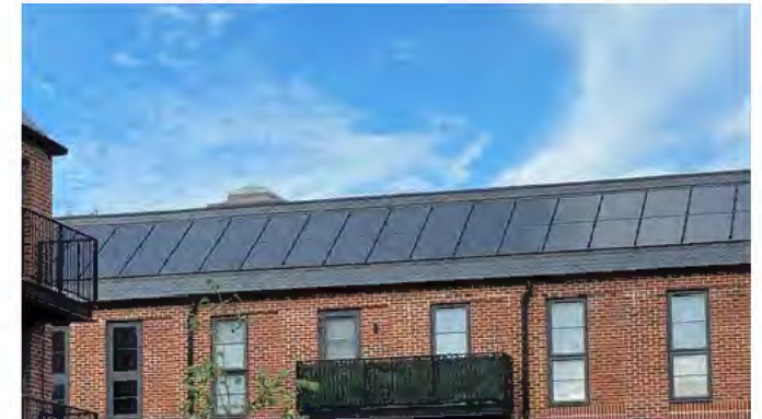
Flush photovoltaic panels incorporated into a roof
