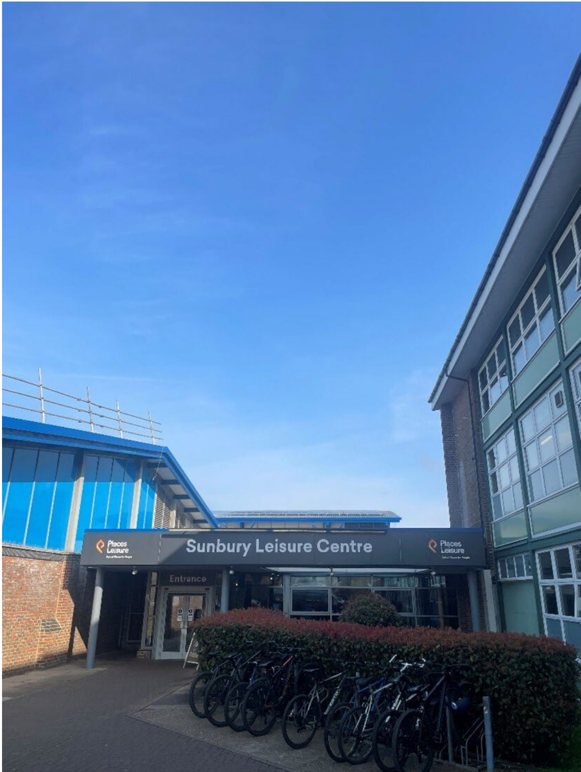
Solar panels power Sunbury Leisure Centre
