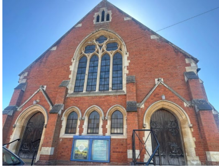
Ashford Congregational Church, Clarendon Road, Ashford, TW15 2QA
