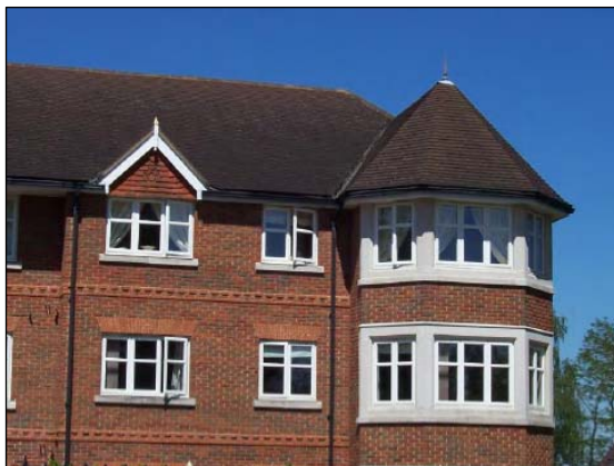
Roof, brick and stone detailing
