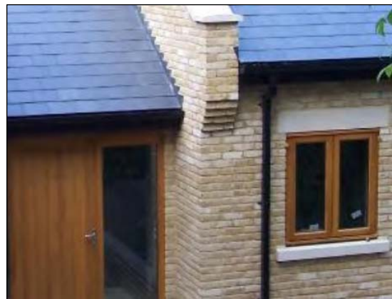
Brick, stone and lead detailing
