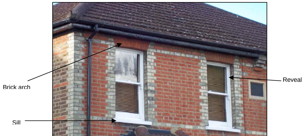
Diagram 9: Components of a window and opening
