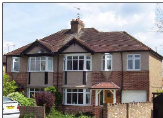
Example of a well designed side extension
