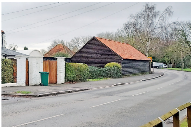
Weatherboarded barn range on the Broadway
