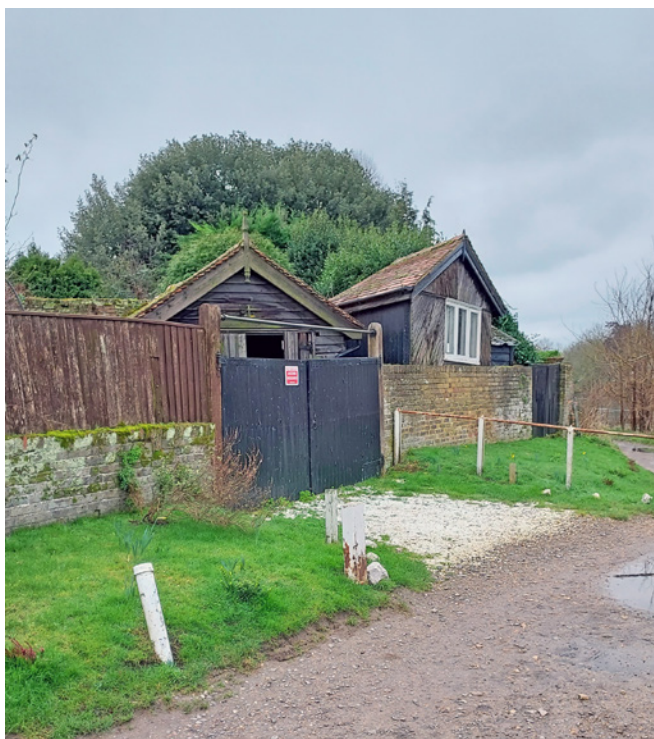
Former boathouses fronting onto Thames Side
