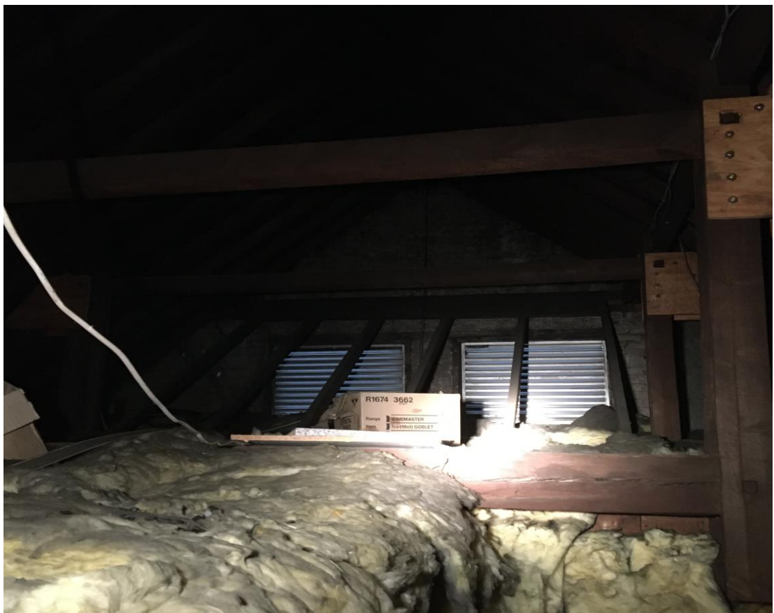
Image EDP 3.6: Internal image of the roof void and vents at the western end of building B1.
