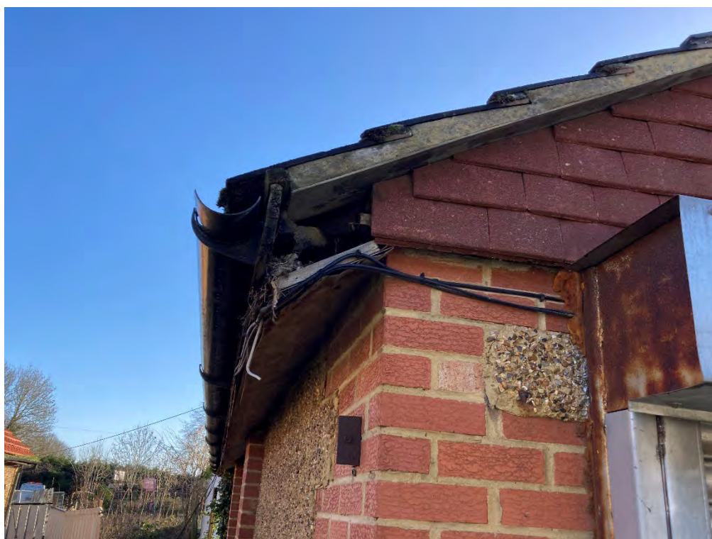
Photograph 18 - Gaps on the corners where the wooden fascia and soffit end
