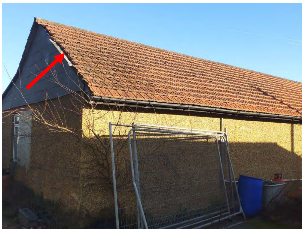
Photograph 10 - B4, with gaps beneath tiles on the western aspect
