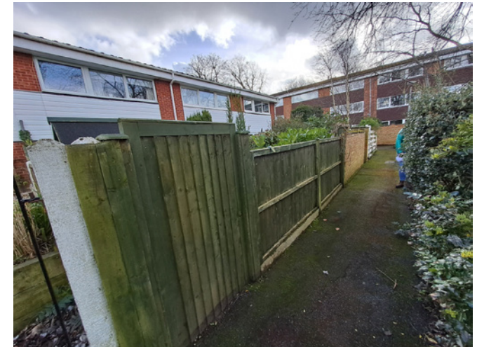
Inappropriate replacement of boundary treatments.
