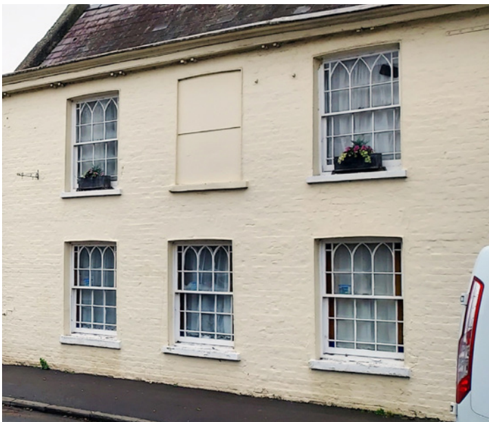
Unusual Gothic windows on Oak Road
