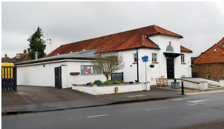
The village hall on the High Street.
